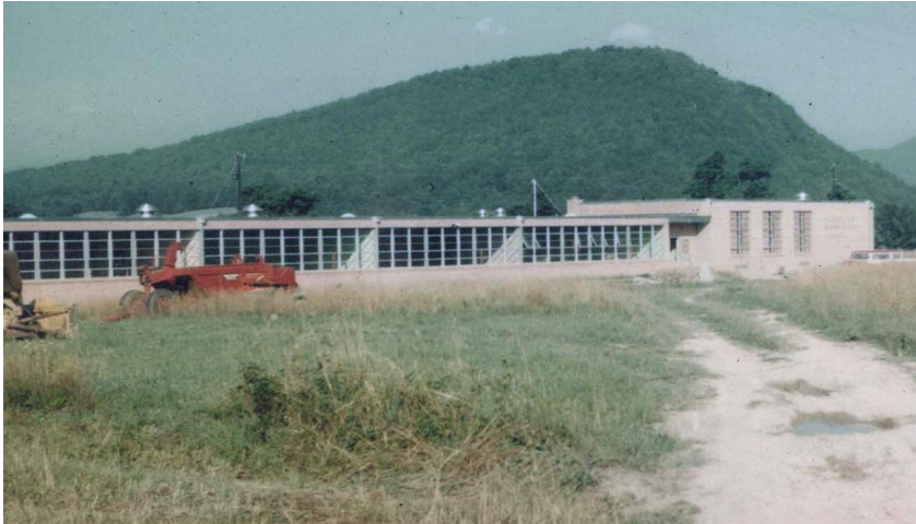
The Fulks Run Elementary School nearing completion in 1961.
